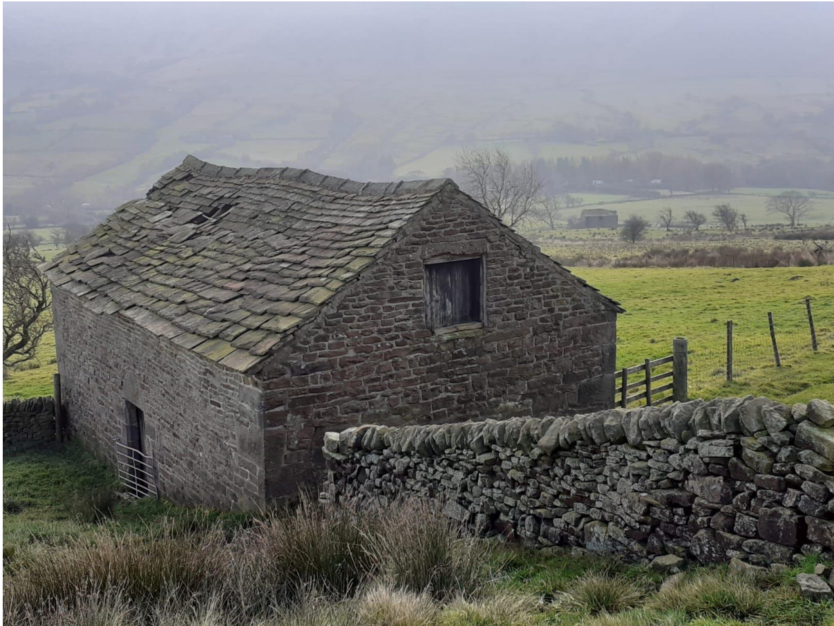
Fig. 3 Field Barn. Edale, Derbyshire. Photo: Andrew Critchlow
